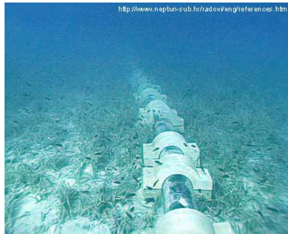
Fig.3. Underwater sewage outlet.
